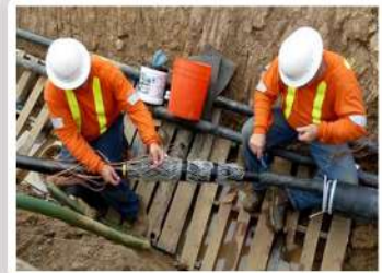
HV Cable Jointers
